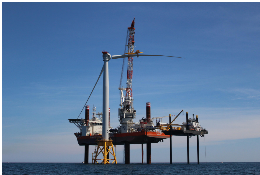
Figure 1. Single blade installation (Image source: RIPR [38]).
